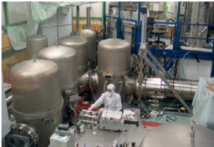
Fig. 3.10 – GEO600 vacuum system.
