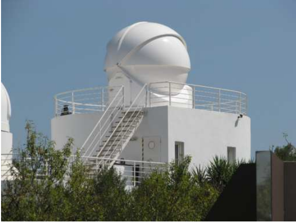
Fig. 3.— The 3.5m Baader Planetarium All Sky dome. The control room is directly below.
