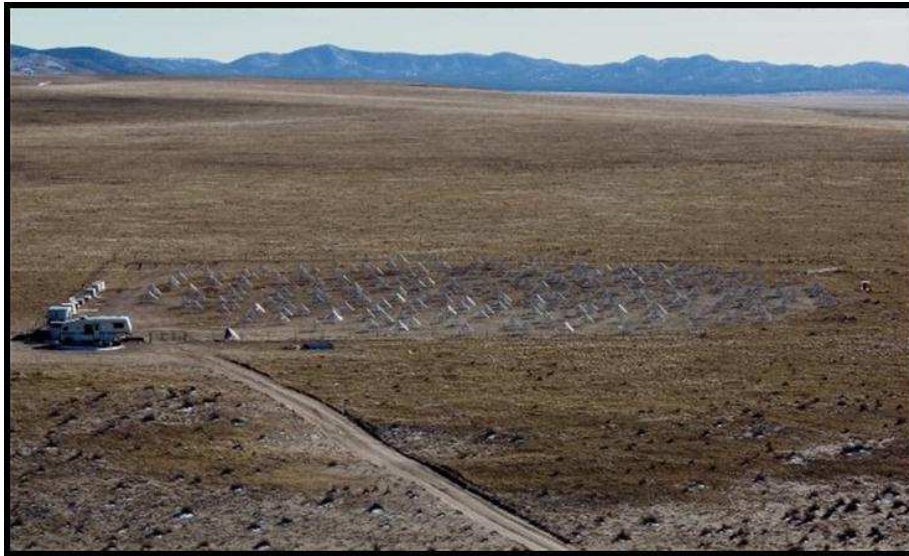
Figure 2: The first station of the LWA, as seen from the EVLA antenna assembly building. The equipment shelter is seen to the left.
