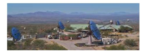
Fig. 1. The four 12m aperture reflectors that constitute the VERITAS Observatory, shown after the relocation of one telescope in the summer of 2009. The reflectors are conveniently distributed around the Administration Building of the Smithsonian's Whipple Observatory in southern Arizona.
