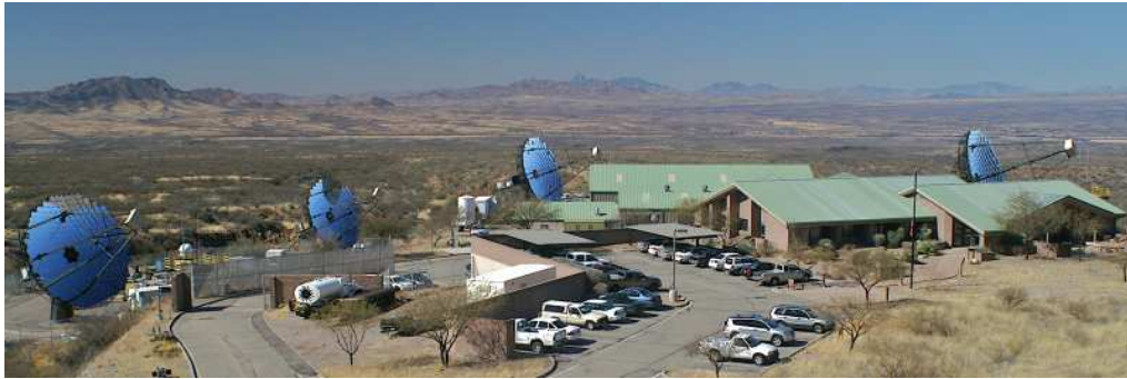
FIGURE 2. The VERITAS observatory, the newest of the third generation IACT observatories, saw first light in April, 2007. Note that VERITAS is in the exact same location as the telescopes shown in Figure 1. Each of the four telescopes has an aperture of 12m (collection area of 106\text{m}^2 ) and a camera with 499 pixels.
