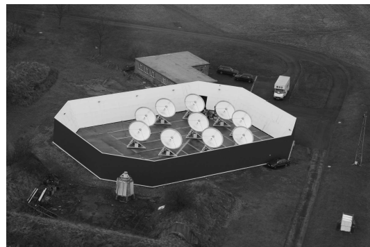
Figure 3. SA from the south east. The correlator is in the building behind. The enclosure floor is now covered in aluminium.
