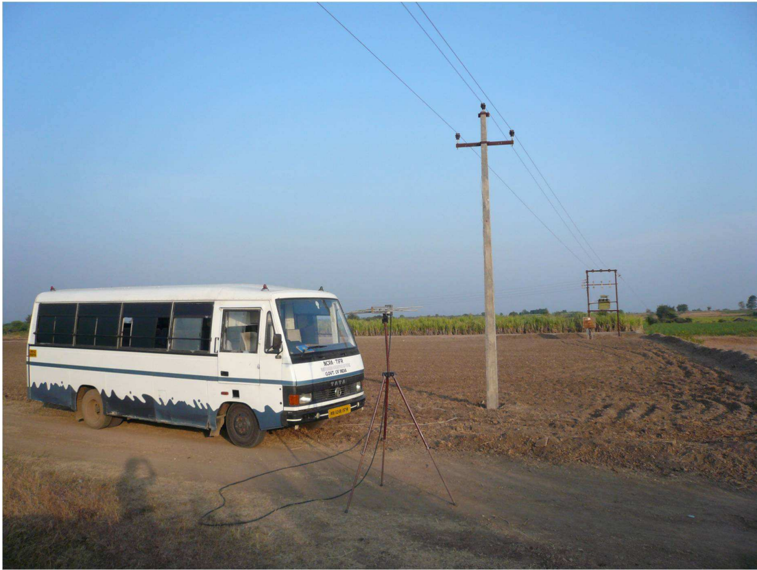
FIGURE 5. RFI localization setup. Power lines are thought to be the primary cause of broadband interference.
