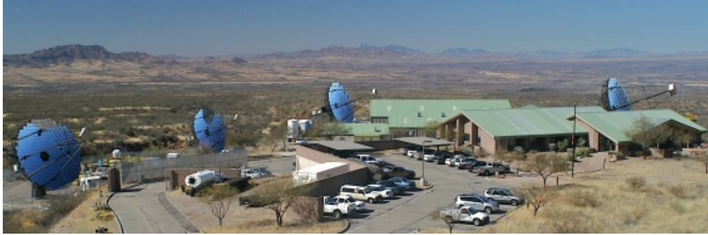
Figure 32. – The VERITAS site [76].
