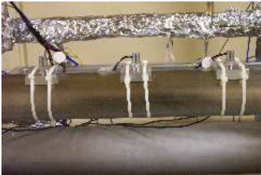
Figure 6: Zoom on 3 sensors installed on top of the C-band structure tested at KEK's main Linac.
