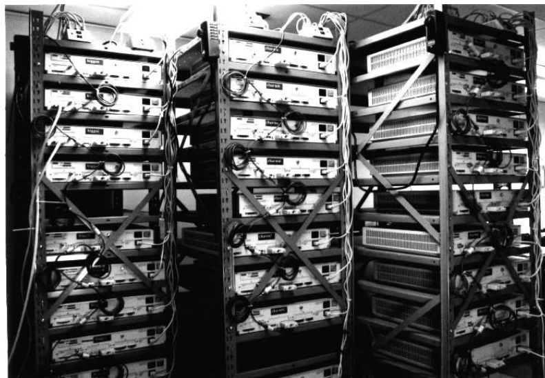
Fig. 2. Rack mounted workstations filtering data; a very cost effective means of computing. A pair of 10 tape Exabyte EXB-10 autoloaders provides an input buffer of over 40 gigabytes. Ethernet distributes events. These particular workstations are DECstation 5000/200s with MIPS R3000 CPUs. Other current possibilities include the Hewlett Packard-Apollo 9000/705, the DECstation 5000/25, the Silicon Graphics Indigo, the IBM RS/6000-320H, and the Sun SPARCstation 2. Running your own benchmarks and comparison shopping is often useful.
