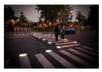
**Fig. 6** Newly installed lighting system in Candia, Quebec, Canada, for improving intersection traffic safety. The image is adopted with permission from the Ville de Candiac [Source].
