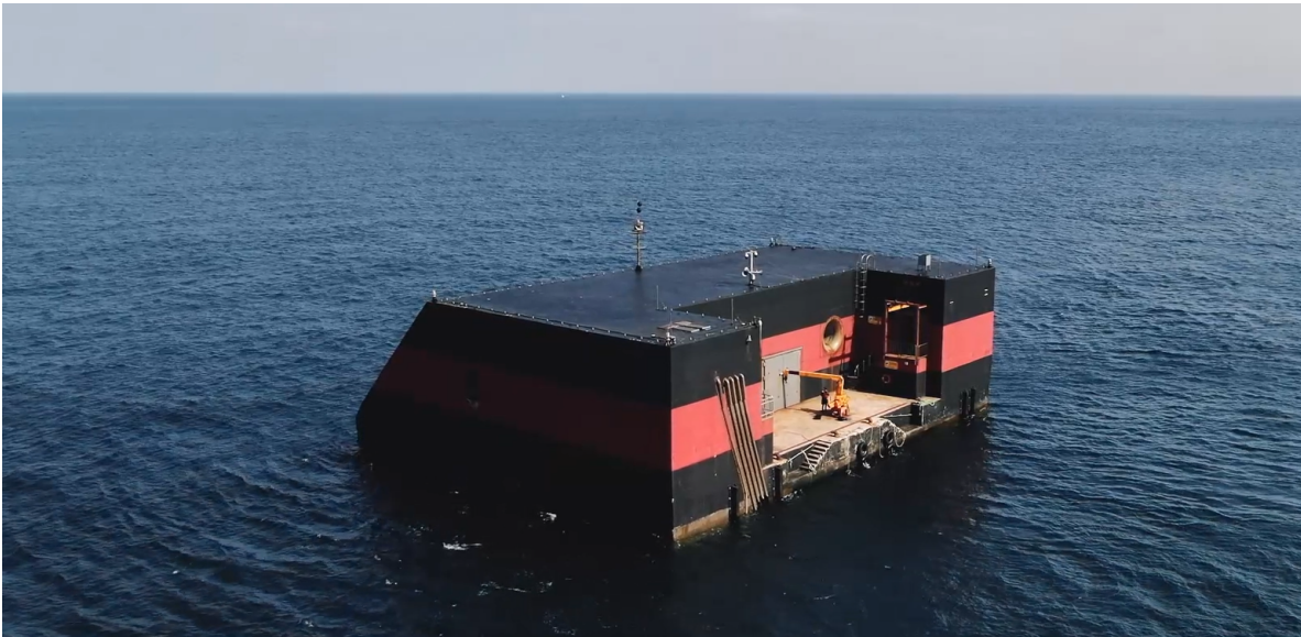
Figure 1: 500kW OWC-WEC at Yongsoo, Jeju, South Korea.
