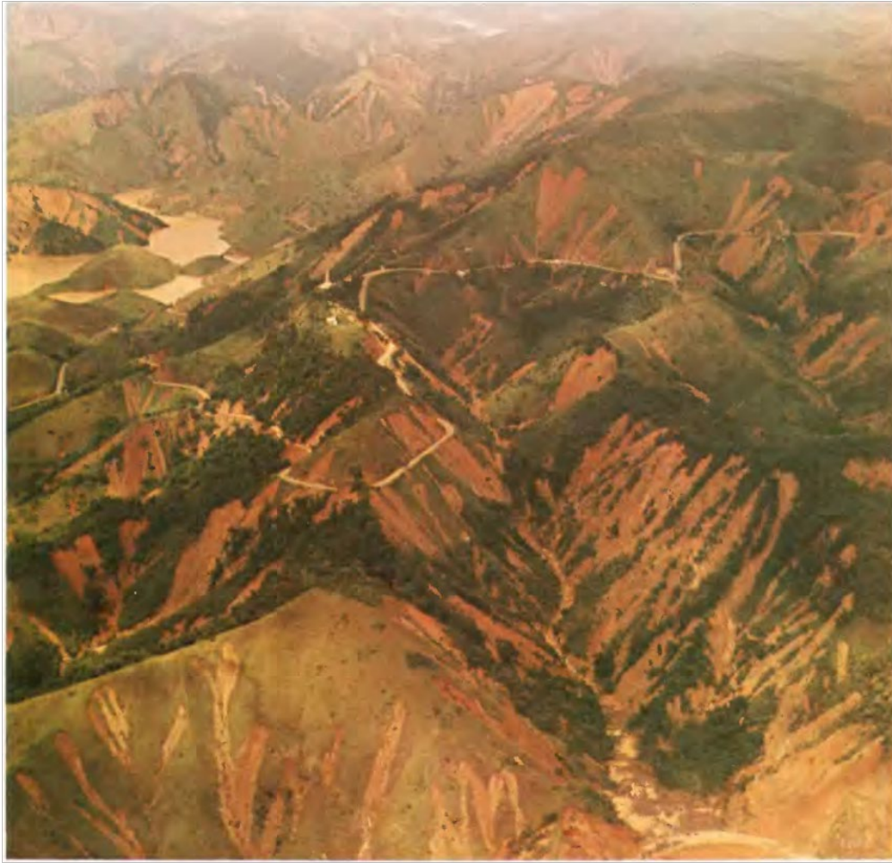
Figure 4 Landslides in the area of the upper part of the old road that crosses the escarpment Serra das Araras-RJ.
