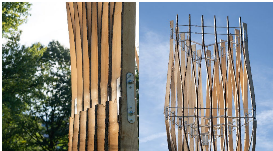
Fig 15 Details of the UnLog Tower : finger joint splice connection (left) and robotically kerfed logs stretched along a thread rod (right), photos by Cynthia Kuo.
