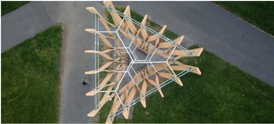
Fig 9 Reciprocally framed tube steel in the UnLog Tower , photo by Cynthia Kuo.
