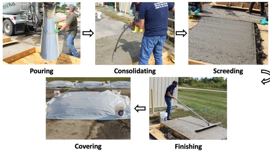
Figure 1. Portland cement concrete casting.
