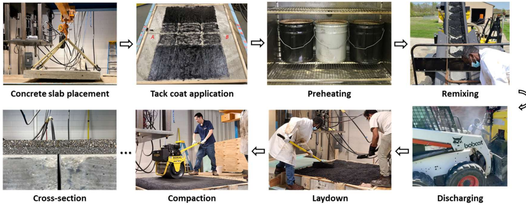
Figure 3. Test pavement construction.
