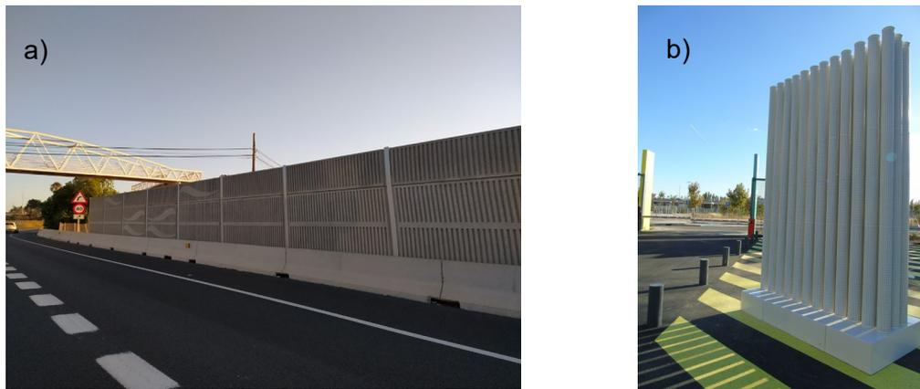
Figure 1. a) photograph of a traditional continuous noise barrier; b) photograph of a noise barrier based on sonic crystals concept.
