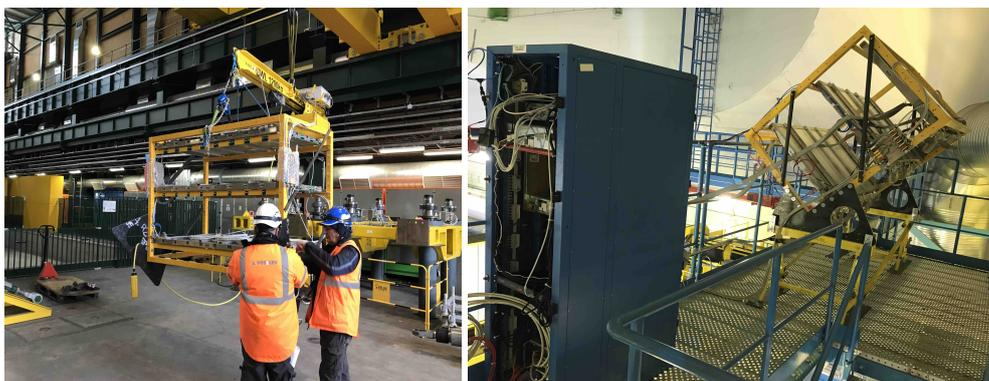
**Figure 3:** (left) A picture captures the moment as proANUBIS is lifted by a crane with the help of ATLAS technical coordination on the surface of SX15 at point-1 of CERN and being lowered through the ATLAS PX14 access shaft. (right) Picture showcases the installation of proANUBIS at its intended position level-12 side-A of ATLAS underground cavern, as seen along with the Data Acquisition (DAQ) rack.
