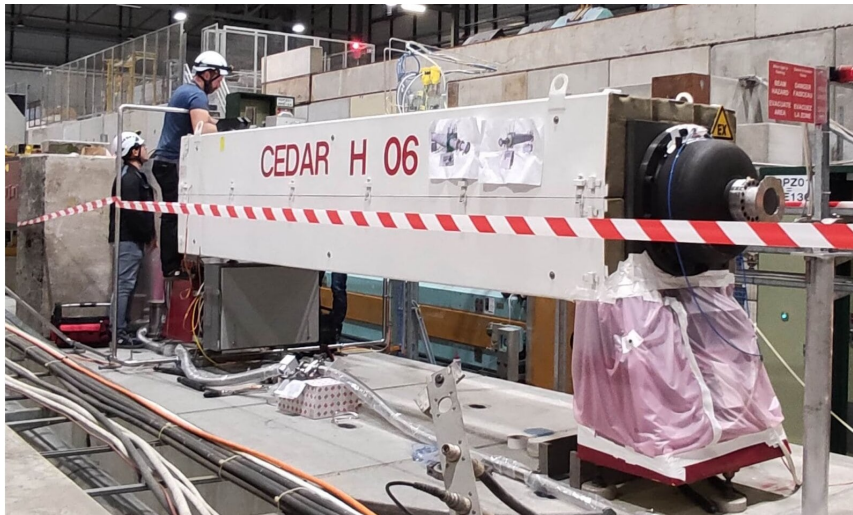
Figure 3. CEDAR-H installed at the H6 beamline at the CERN SPS .
