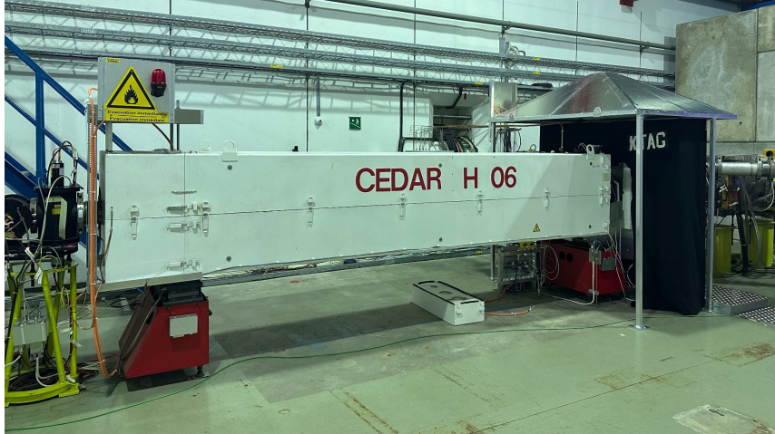
Figure 5. CEDAR-H installed in the NA62 beamline, with the flammable gas safety hoods on both the downstream end (left) and the upstream end above the black KTAG enclosure (right). The XY motors are found in the red foot at the downstream end (left).
