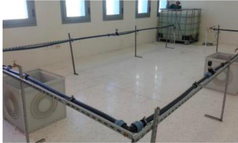
Figure 2: EARNPIPE testbed is developed with polyethylene pipes (Karray et al., 2016)
