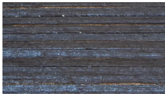
Fig. 1: A photo of the AFP-manufacture structure shows gaps and overlaps between the composite tows.
