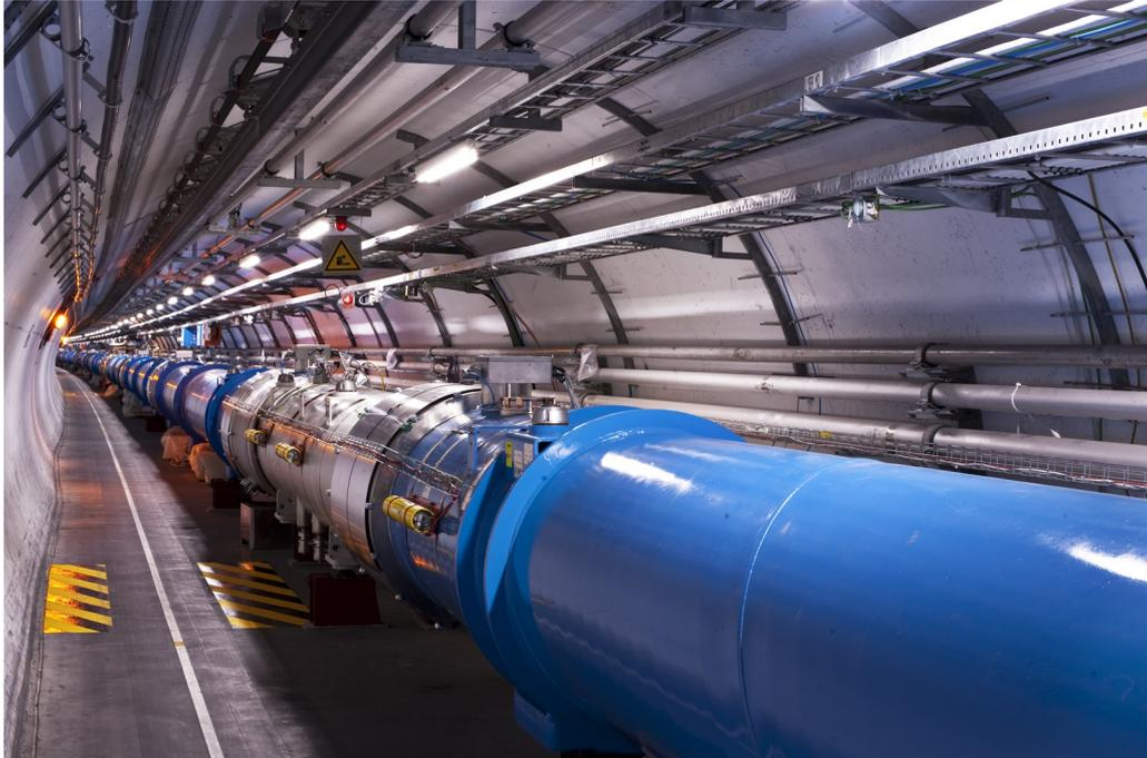
**Figure 3:** Dipole magnets, which are painted blue inside the LHC tunnel. The small yellow sign hanging from the ceiling indicates a oxygen deficiency risk in case of a gas leak. From Ref.[16]
