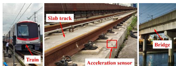
Fig. 7. Placement of acceleration sensors.
