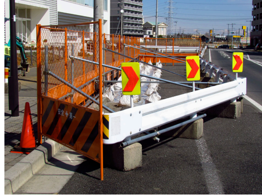
Figure 15: Photo of decontamination work at the same place in Fig. 9.
