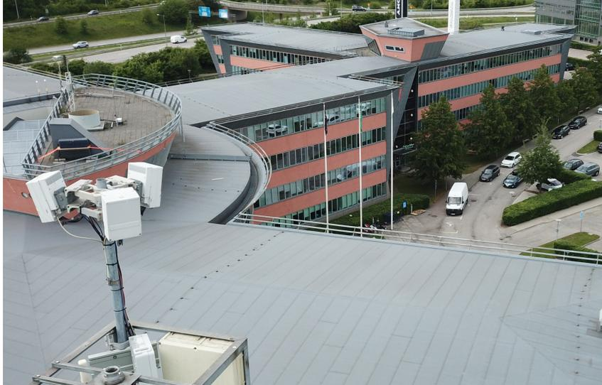
Fig. 2. The tower BS site, with three Ericsson AIR 5322 Antenna Integrated Radio unit mounted to cover the surroundings. The unit facing the parking area was the one used during the experiments.
