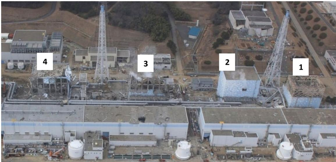
**Fig. 3.** The status of the FDNPP Units 1, 2, 3, and 4 after the accident, retrieved and modified from the American Nuclear Society schematic [56]. The hydrogen explosions destroyed the reactor buildings of Units 1, 3, and 4. Unit-4 reactor building experienced a hydrogen explosion due to the backflow of hydrogen from Unit 3 via the interconnected ventilation system [28].
