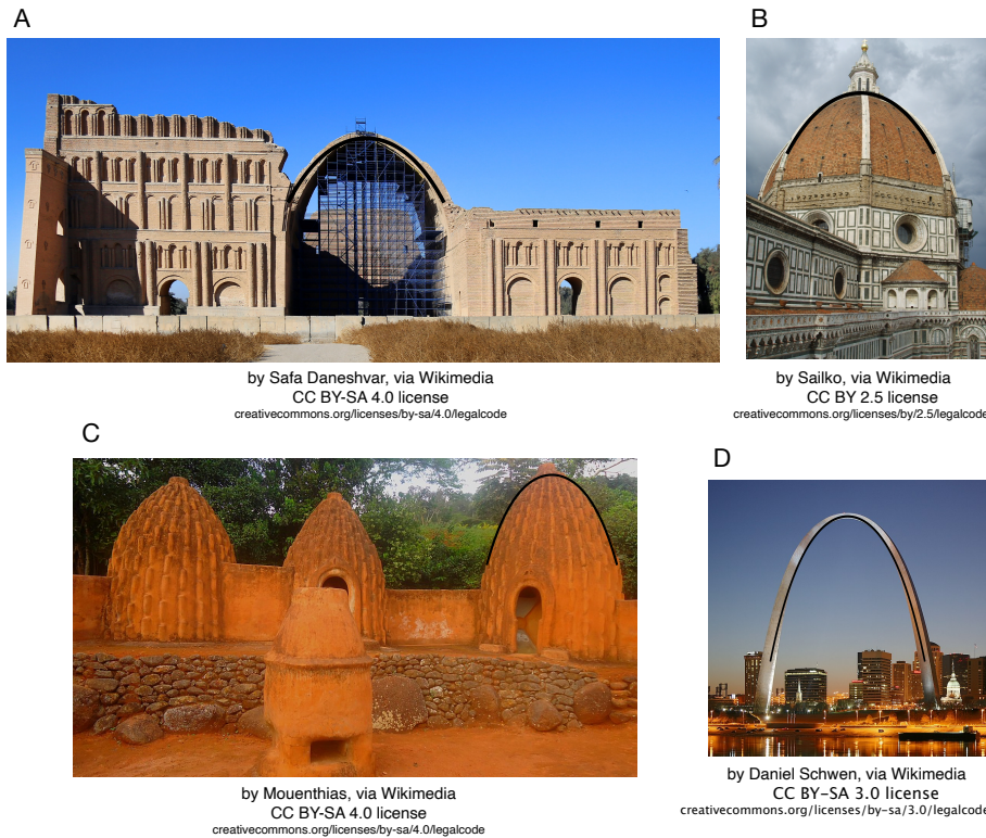
Figure 4 Examples of catenaries and catenary domes in architecture. A: The Arch of Ctesiphon, a Persian monument in present-day Iraq, about 1500 years old. B: The dome of the cathedral of Florence, built between 1296 and 1436. C: Traditional houses of the Musgum people in Cameroon. D: The Gateway Arch in St. Louis. It is a weighted catenary. The black curves are catenaries in panels A–C, and a weighted catenary in panel D.
