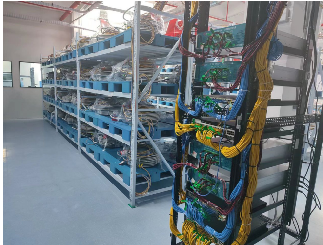
(b) Shelf with UWBoxes in the testing room in Kunshan.
