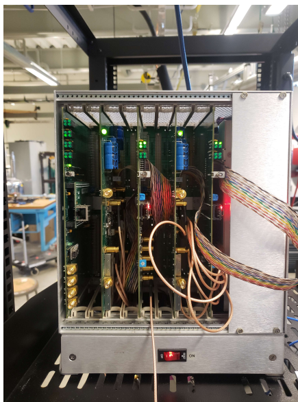
(b) LANL System in VME Crate
