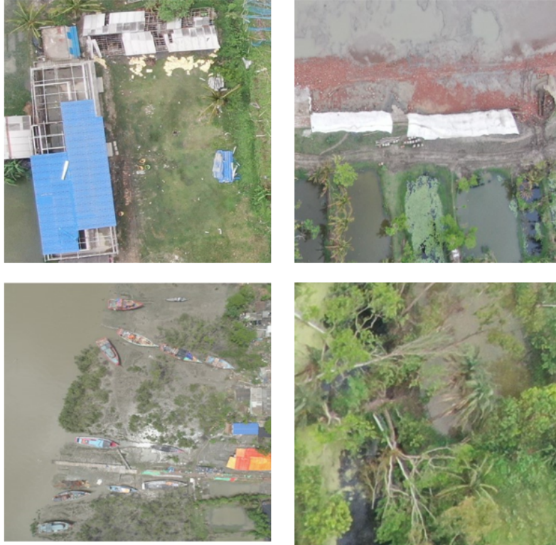
Figure 2: Damages captured by UAVs in West Bengal: damaged building, damaged Jetty, uprooted trees, damaged embankment (anti-clockwise from top corner)
