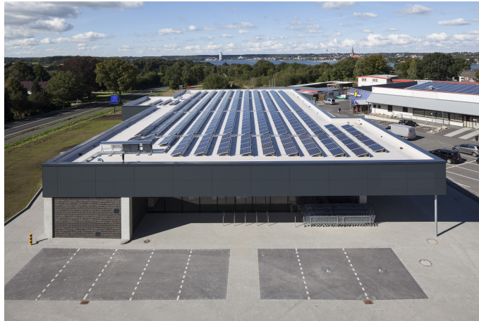
Figure 1: Example of PV system within the portfolio.
