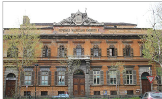
Figure 7.1 Umberto I, Mauriziano hospital in Turin.
