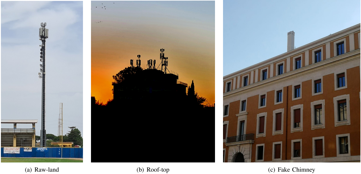
Fig. 4. Main types of cellular towers.
