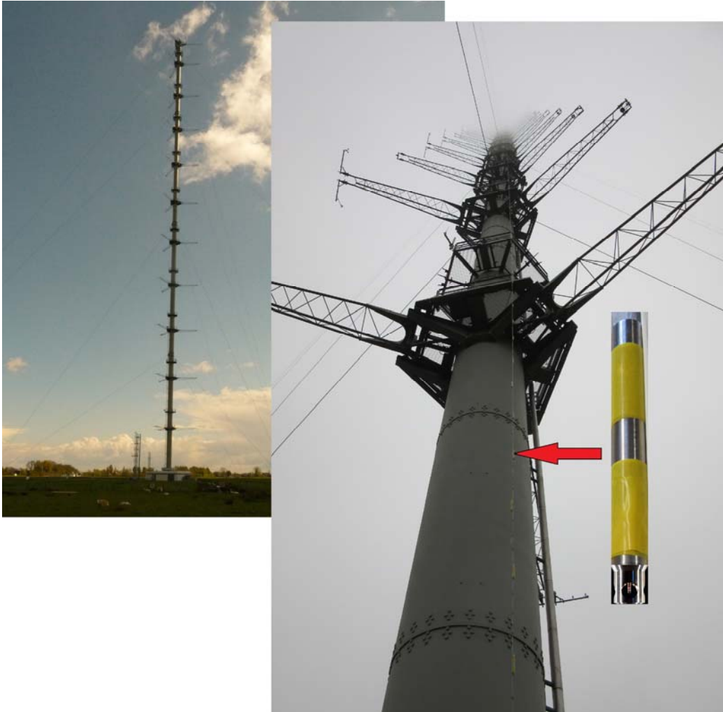
Fig. 1. View from the north of the entire 213-m tall KNMI-mast in Cabauw in summer, and, in the foreground, from the south and from below in autumn-fog with lower end of temperature T-sensor cable suspended along-side (the red arrow points at a 0.18 m long T-sensor).
