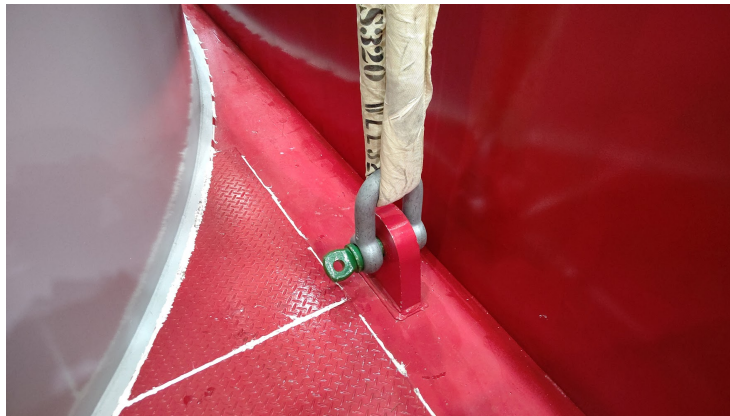
Figure 6: A shackle tied to the detector. Four shackles are used to lift the detector.
