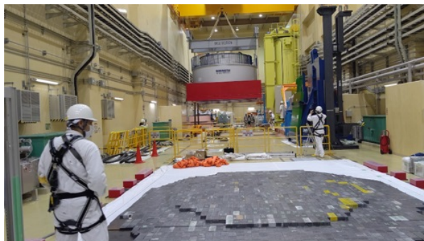
Figure 3: Gamma-ray shielding layers consisting of iron plates and lead blocks. The 70 tonne detector with Gd-LS and LS was transported by a crane and installed on the shielding layers.
