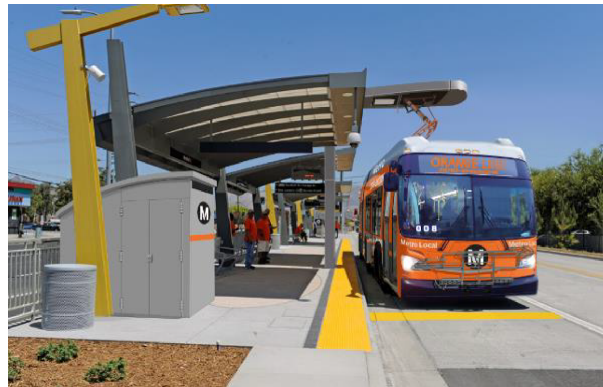
Figure 1- Orange line electric bus equipped with SAE3105-1 charging station [6].
