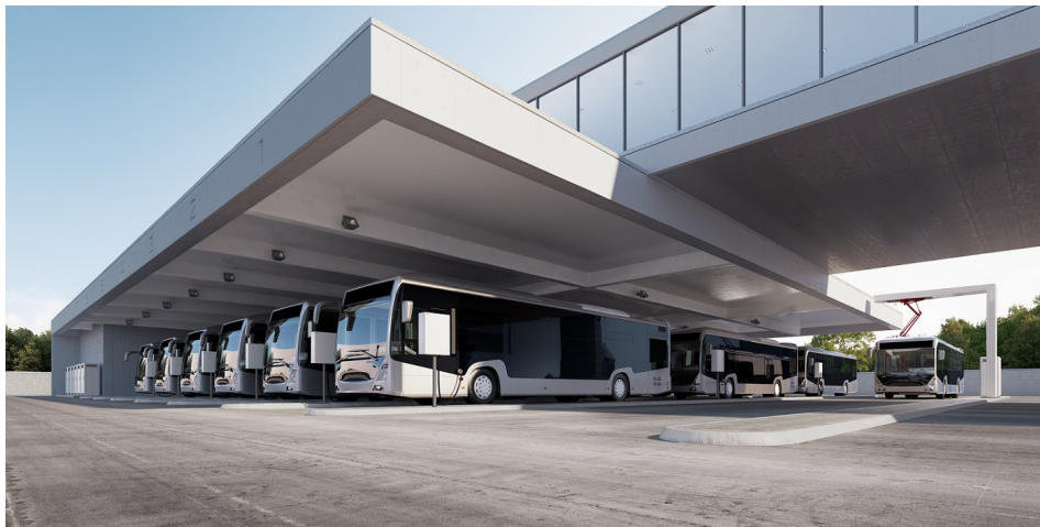
Figure 5- ABB depot charging station, purposed for overnight charging [11].
