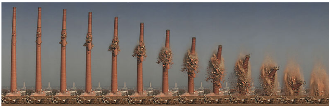
Figure 14. Time sequence of controlled demolition blasting of a chimney at the former Henninger brewery in Frankfurt am Main, Germany, Sachsenhausen (Source: Heptagon, Wikimedia Commons).
