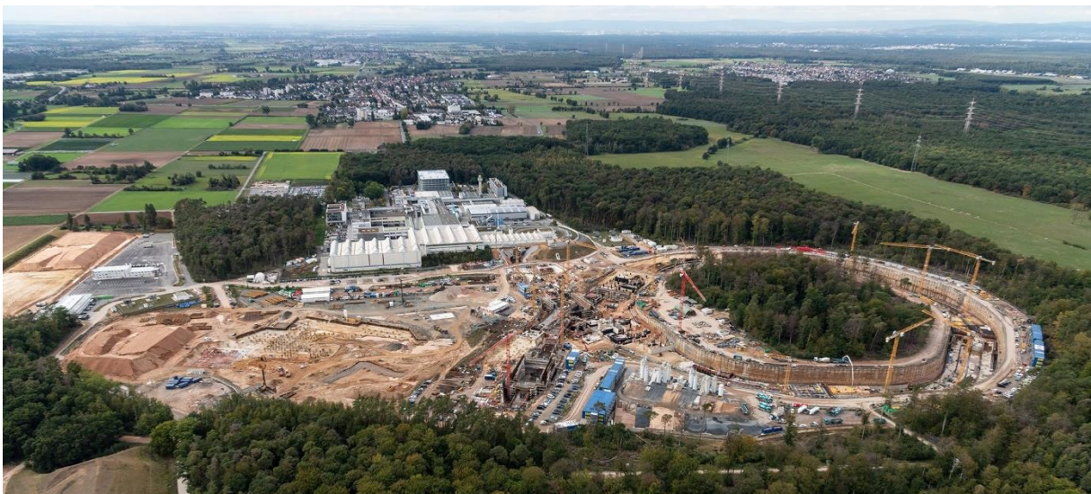
Fig.18: Photo of the FAIR construction site from September 2020 [57].
