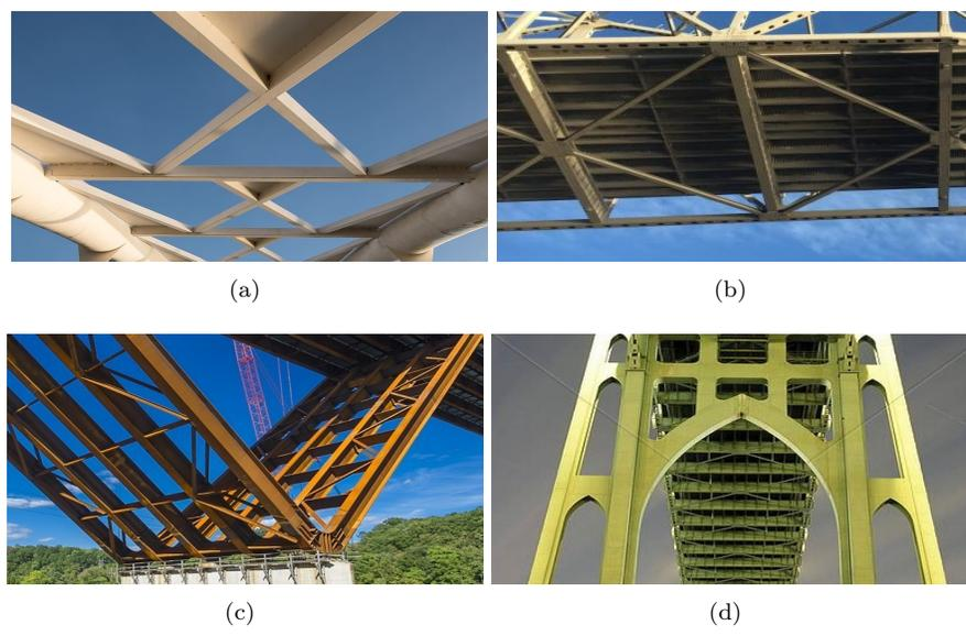
Figure 2: The typical steel bridges structure: (a) *cross shape*, (b) *K-Shape*, (c) *L-Shape*, (d) and *combination of shapes*
