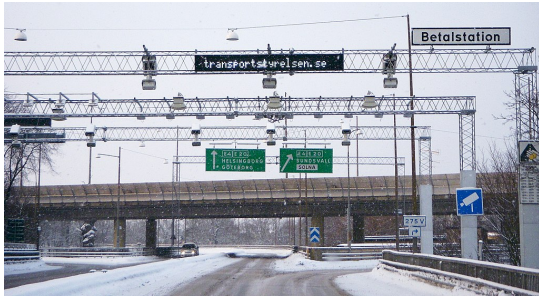
Figure 2: An example of a laser-based traffic sensor used in this paper; photograph by Holger Ellgaard, distributed under a CC BY-SA 3.0 license.
