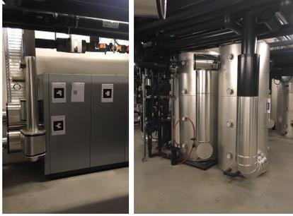
**Figure 5:** Experimental facility with heat pump and water storage tanks [9]
