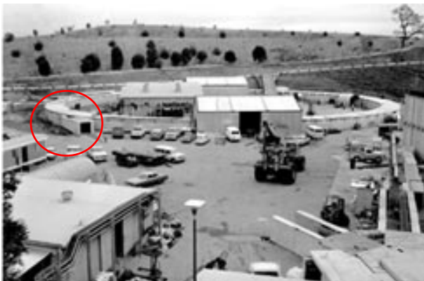
Figure 3. The SPEAR ring under construction at SLAC.
