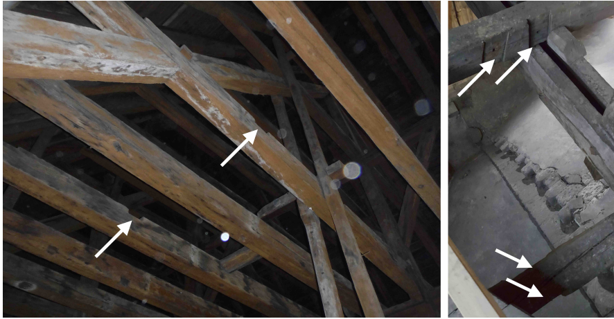
Figure 2: Notches indicating the reuse of ancient wooden beams.
