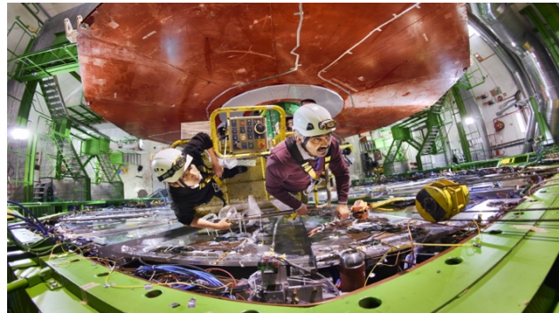
Figure 2. A picture taken during the removal of one of the RE+4 supermodules.
