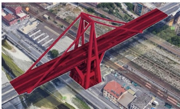
Fig. 2: Collapsed stack 9 balanced system highlighted in red [10]
