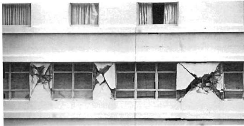
Figure 31. Damage imposed on the short columns and shear wall components in Northridge earthquake [23]
