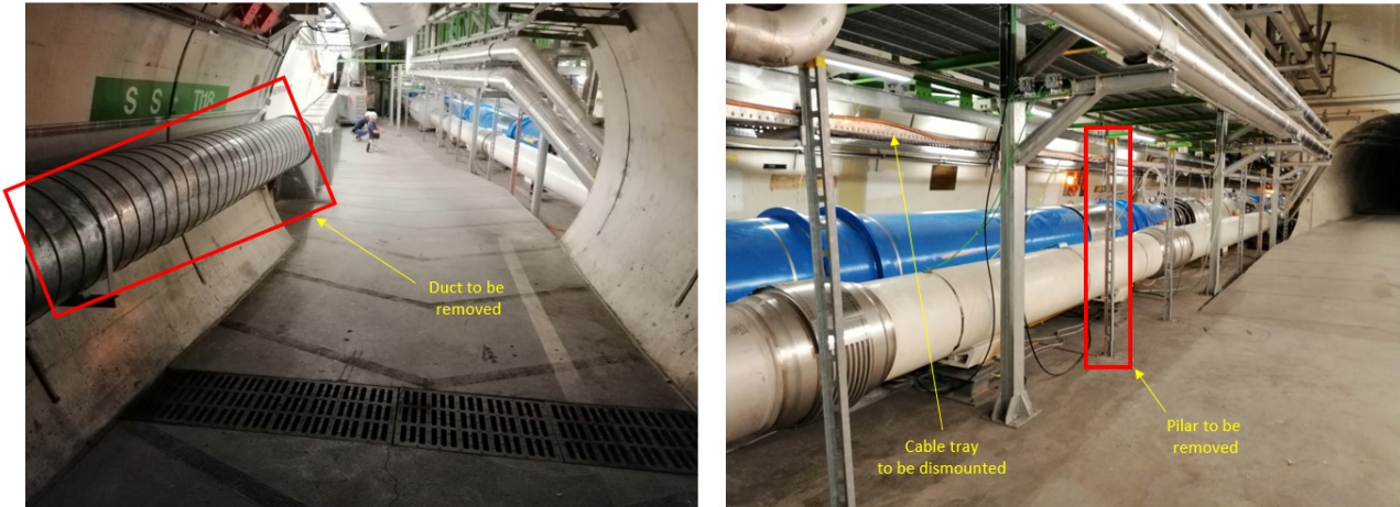
Figure 17: Activities to be carried out for the ventilation duct removal
