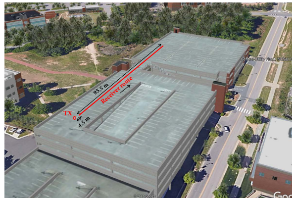
Fig. 2: Outdoor measurement setup at the top floor of a multi-story car park, Centennial Campus, North Carolina State University.
