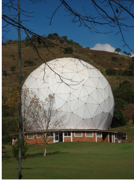
Figure 2: The dome protecting Itapetinga 13.4 m radio telescope at Atibaia (Brazil) is an example of discretization of a curved surface by a set of juxtaposed plane polygons.
