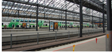
Fig. 2. Photo of the railway station (STA) measurement site.
