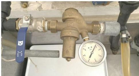
**Figure 2. Shut-off valve, pressure regulator and pressure sensor (manometer).**
